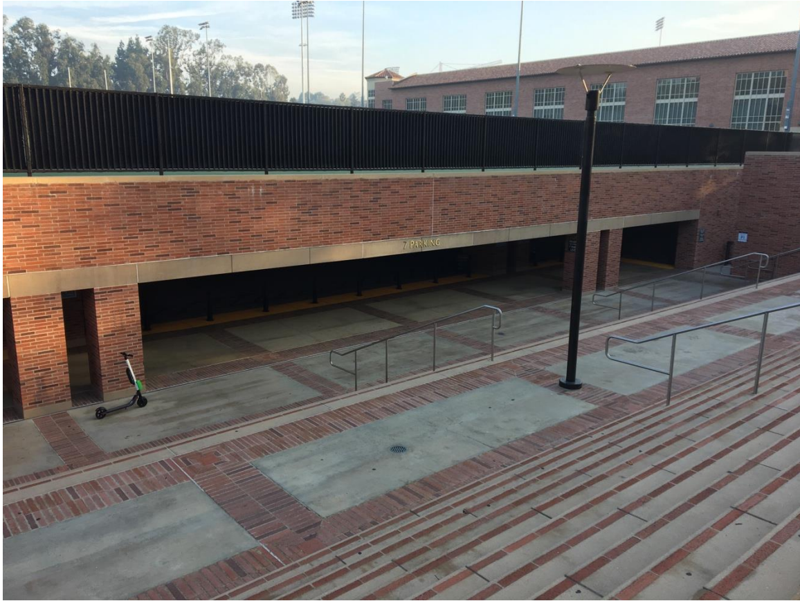
Figure 11. Parking Lot 7. Image of underground entrance of Parking Lot 7.
