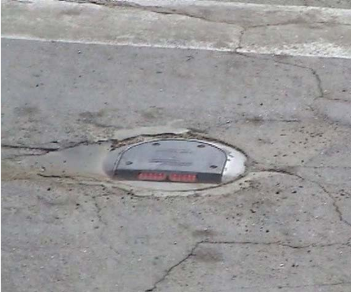
Figure 16: A close-up of one of the embedded lights as it is firing.
