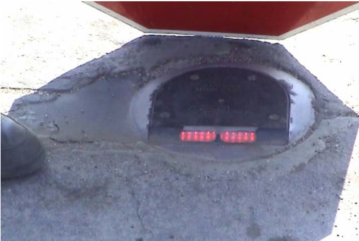
Figure 17: The conspicuousness of the firing light improves markedly when not in direct sunlight.
