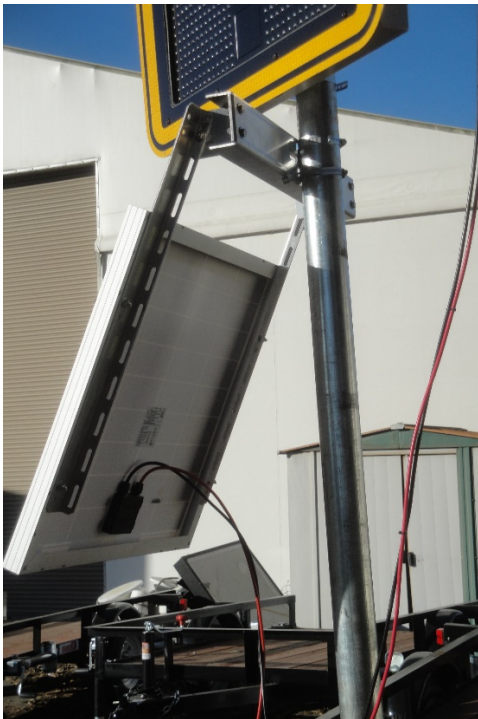
Figure 4.6 VSA sign and solar panel wire connection
