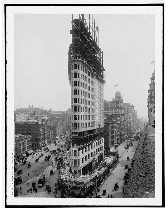
Fig. 5. Flatiron Building under construction, New York, N.Y., c. 1902. Photo credit: Detroit Publishing. Library of Congress Prints and Photographs Division.
