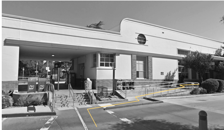
Figure 9.11: The ramp that users need to negotiate, with a highlighted yellow path indicating the route.
