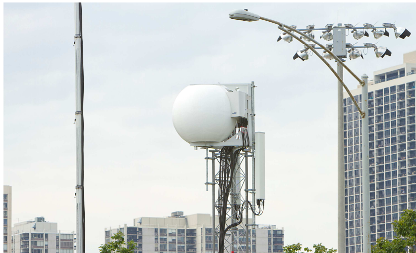
Figure 5-1: AT&T's Giant Eyeball Antenna (also known as the Luneburg Lens Antenna) [79].
