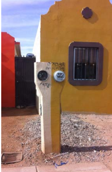
Figure 13. Common location of metering systems in low-income neighborhoods in Mexico. NOTE: The picture shows a metering system on the right, and a void in the place where the missing metering system would be for the house on the left. Photo by the author.
