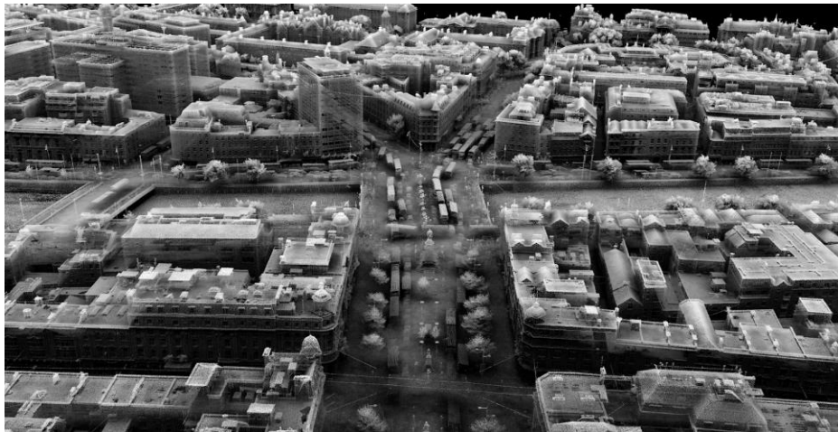
Fig. 10. LiDAR depicting view southwards from the point of The Spire. Digital rendering by Brittney O'Neill and Debra Laefer, 2017.
